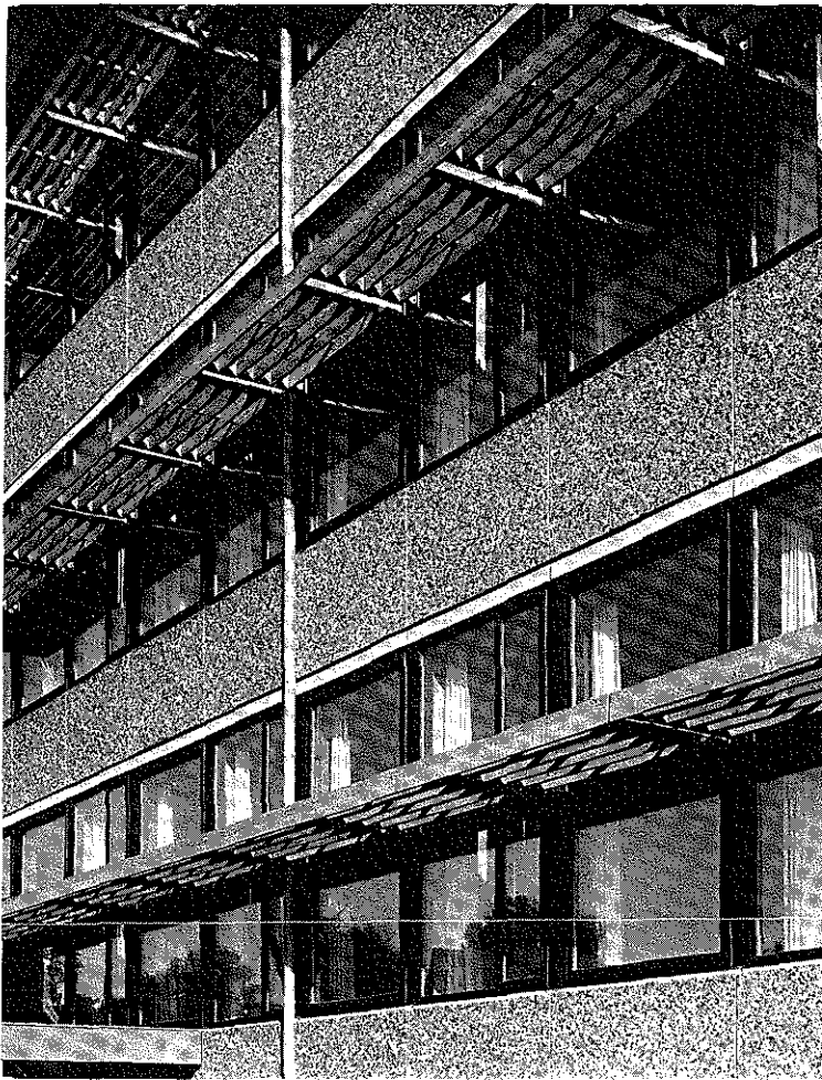
Figur 18.04. Skole med facader af be- tonelementer med frilagte overflader. ★ School with external walls of concrete panels with surfaces of exposed aggregates.
